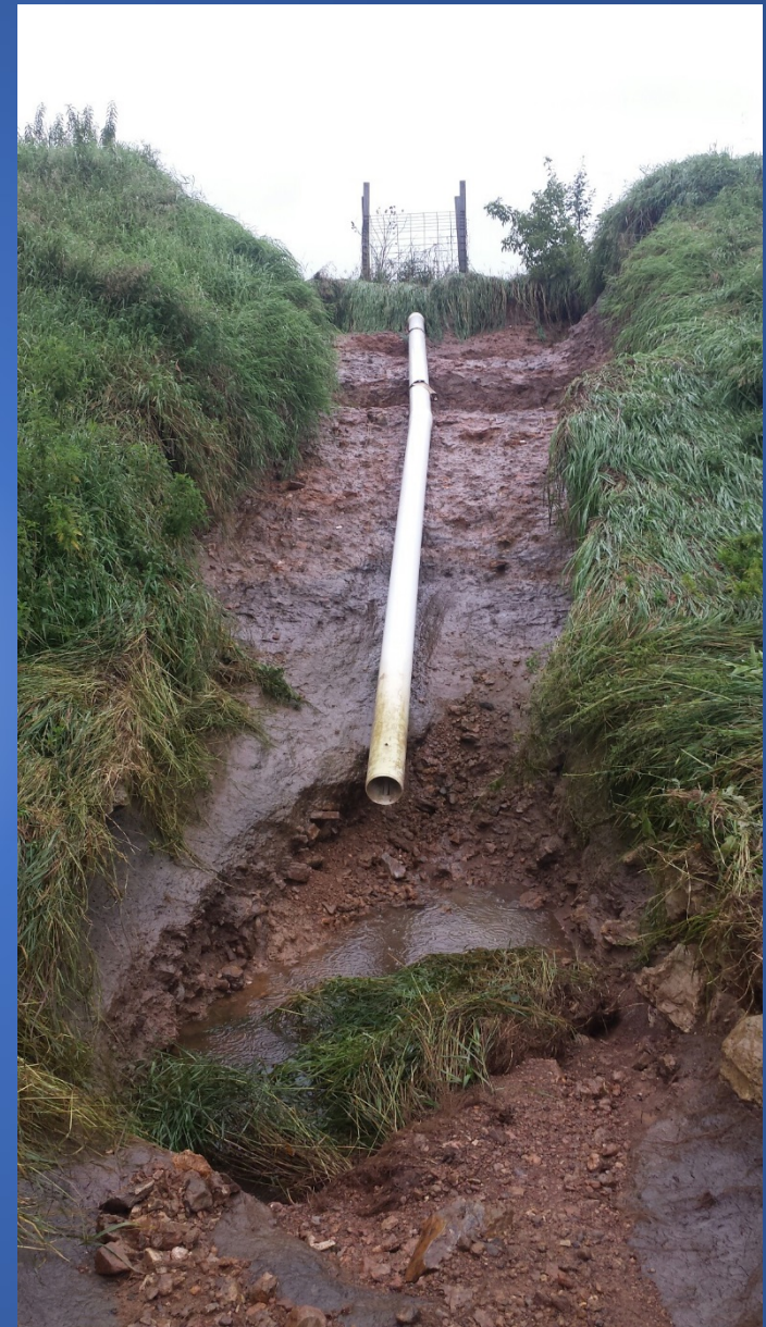
Grade Stabilization Structure
