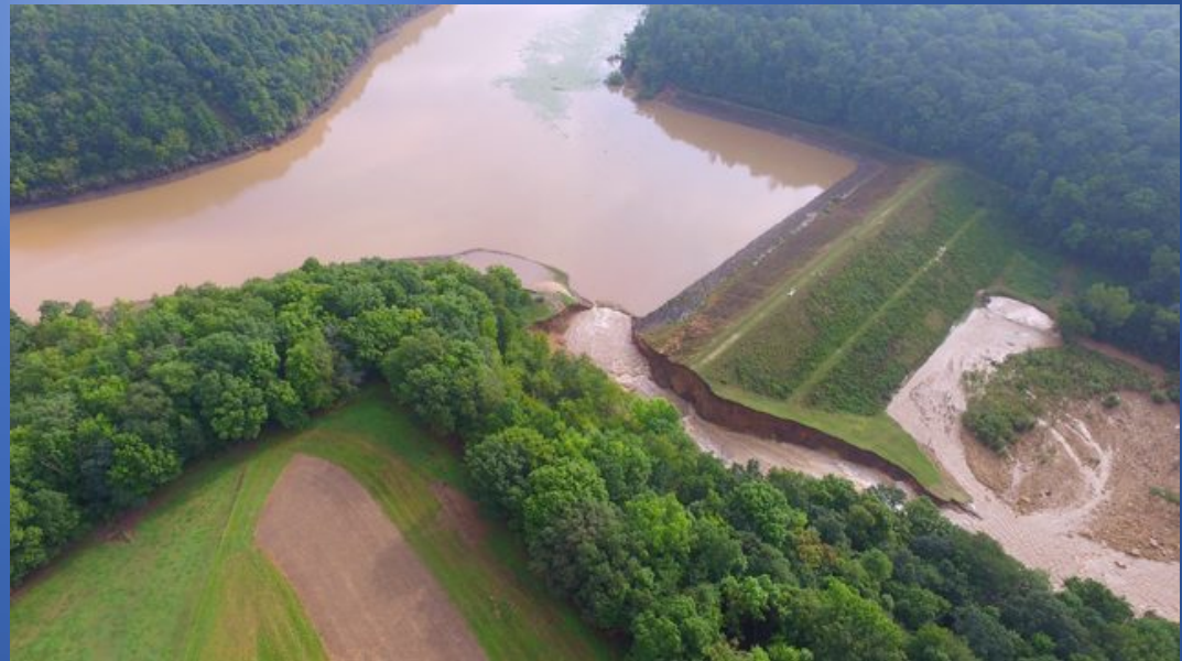
Jersey Valley – Dam Breach – (Kickapoo)
